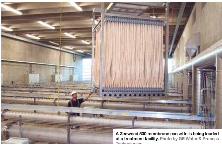
A Zeeweed 500 membrane cassette is being loaded at a treatment facility. Photo by GE Water & Process Technologies
